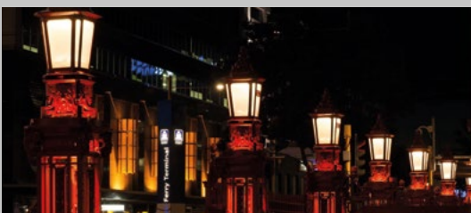
Red Fence Street lighting, NZ
